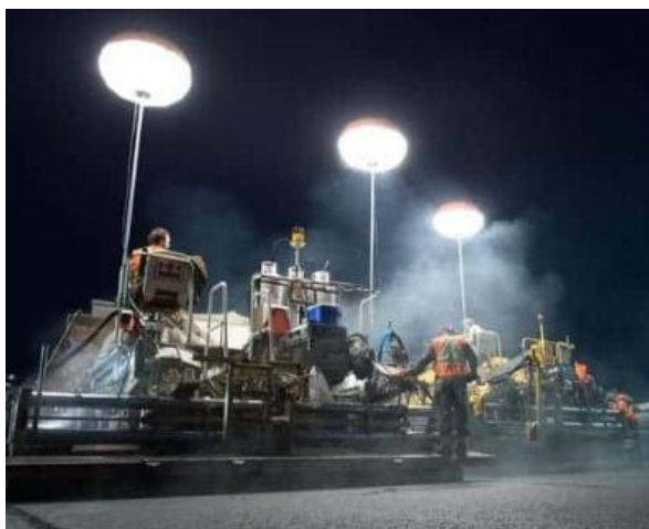
Figure 900 - 1 "Balloon" Type Lighting
