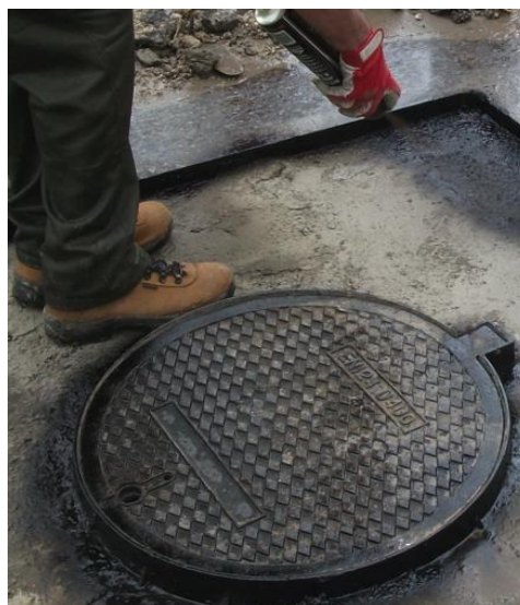
Figure 550- 5 Sealing and Tack Coat
