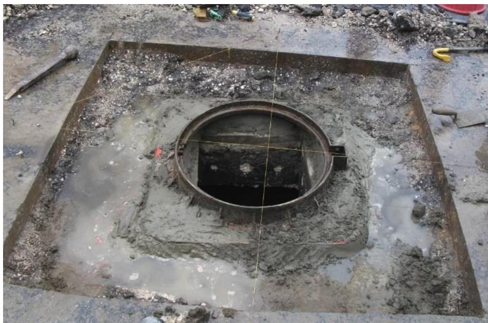
Figure 550- 1 Levelling of the Frame
