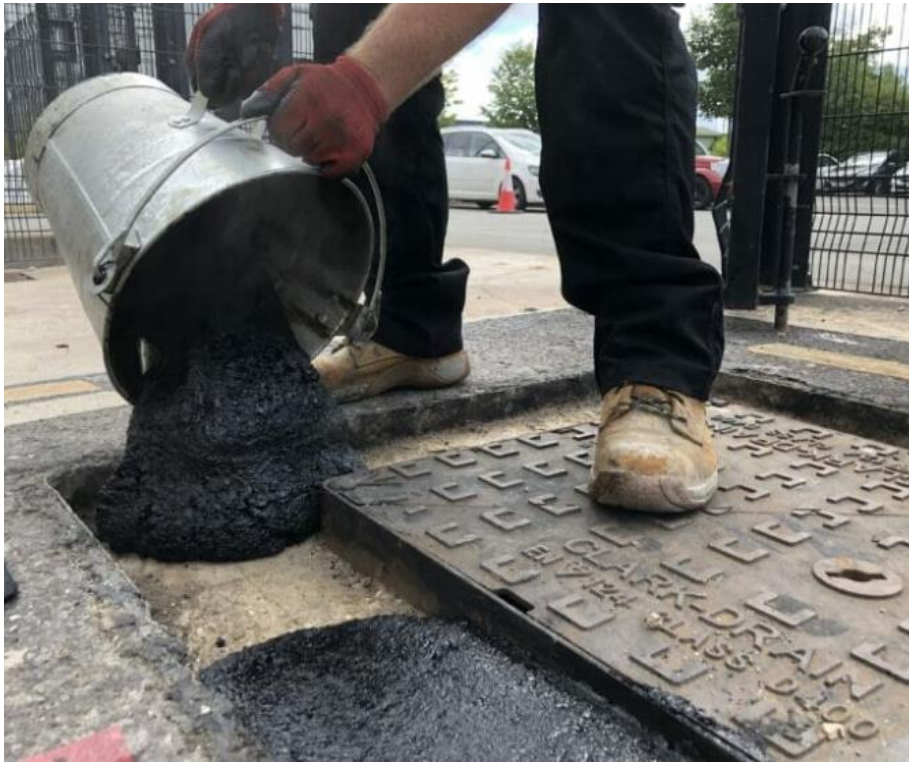
Figure 550- 7 Alternative A – Placing of Hot Material (Mastic)
