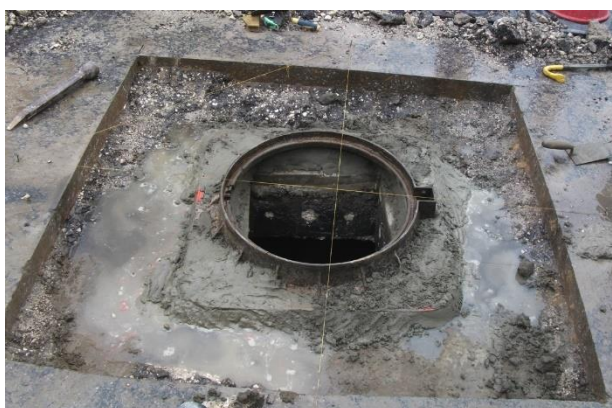
Figure 550- 1 Levelling of the Frame
