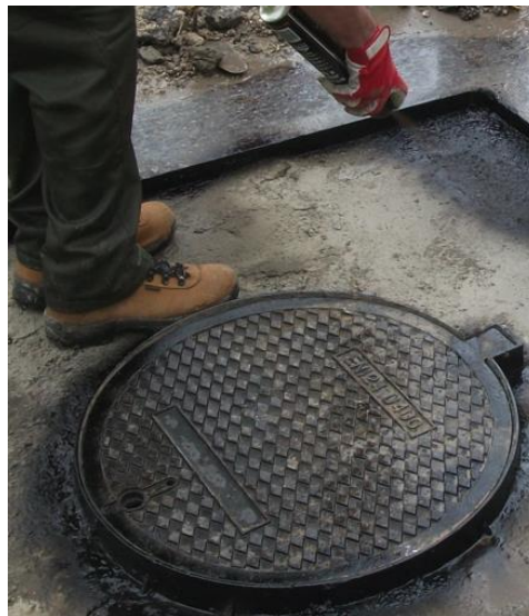
Figure 550- 5 Sealing and Tack Coat
