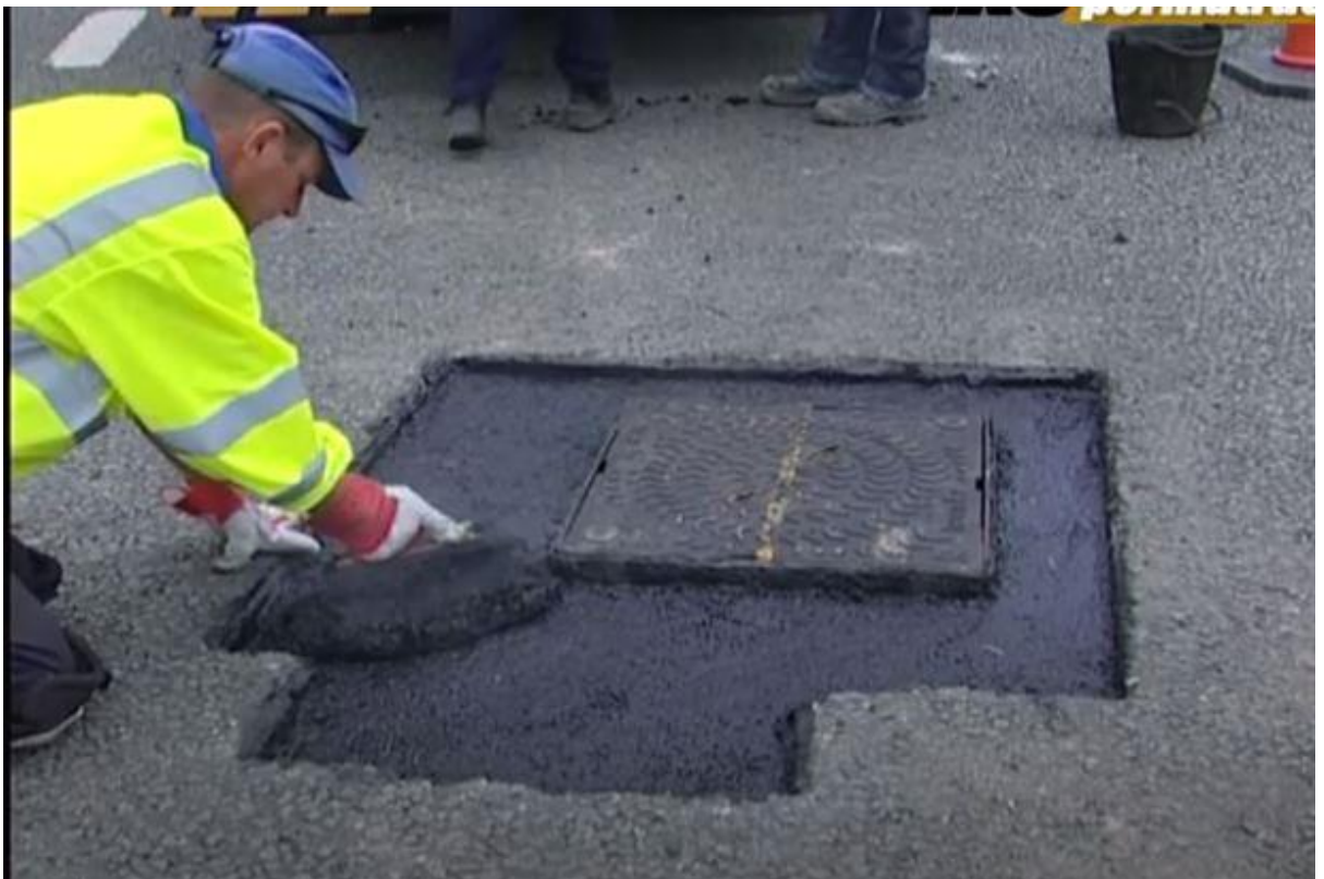
Figure 550- 9 Alternative A – Hand-levelling of Hot Material (Mastic)
