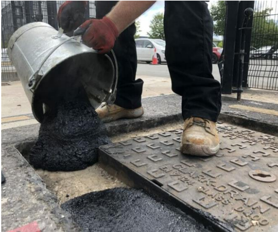
Figure 550- 8 Alternative A – Placing of Hot Material (Mastic)
