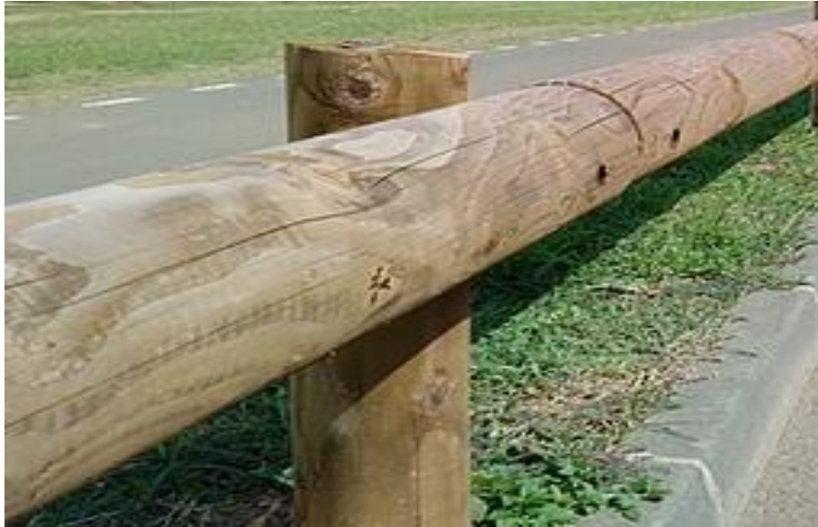
Figure 400 - 5 Timber-clad VRS (Illustrative – Round)
