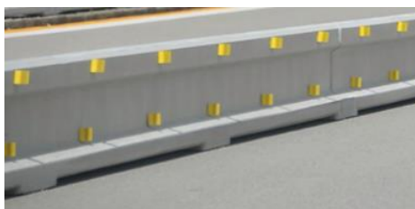
Figure 2: Temporary VRS - Concrete
