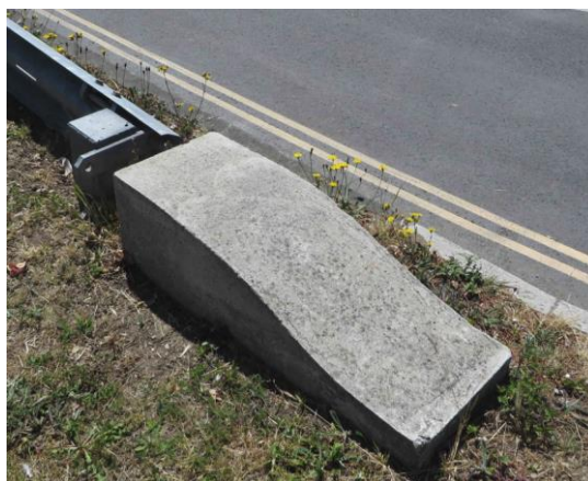
Figure 400 - 2 Terminal Anchorage Concrete Unit
