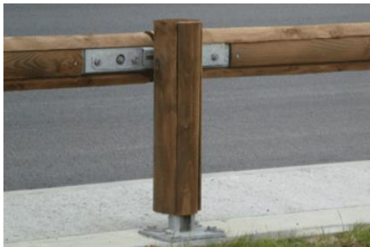
Figure 400 - 6 Cladding at back of exposed members (Illustrative)
