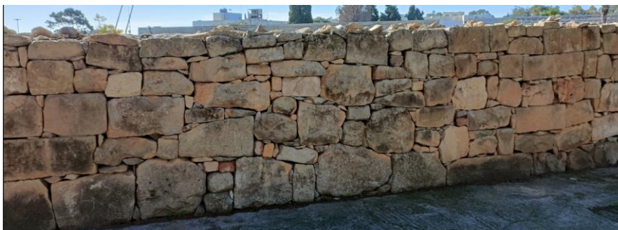
Figure 2400- 1: Dry Rubble Wall (Illustrative)
