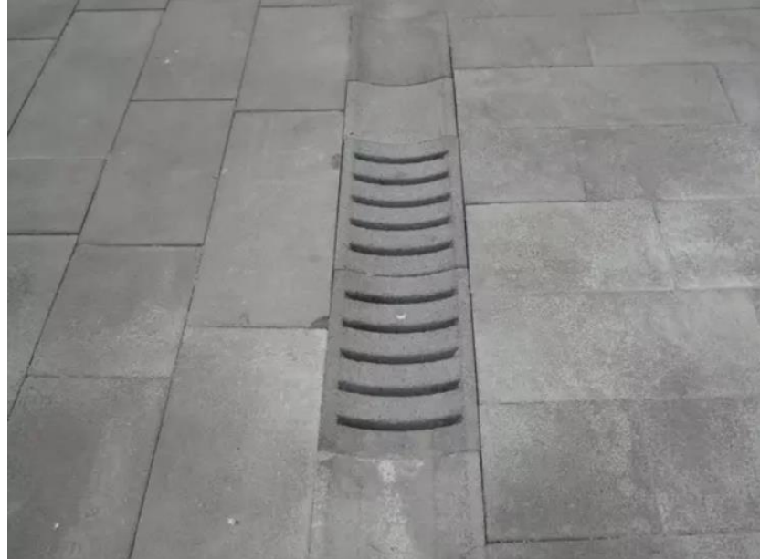
Figure 5 Ancillaries – Lava “Slotted” Drain Channel Units (Illustrative)
