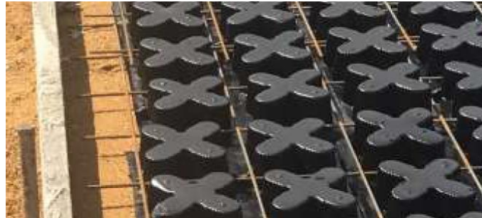
Figure 9 Mesh Reinforcement and Void Formers
