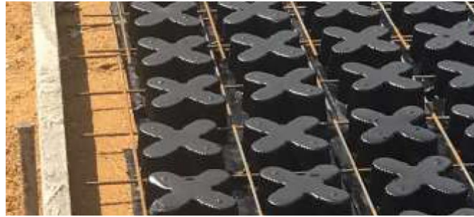
Figure 6 Mesh Reinforcement and Void Formers
